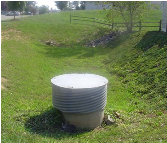
Photo from June 2011 inspection of Extended Detention Pond at 233 Norcroft Terrace.
