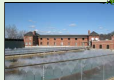
Settling basins remove large and medium particles. Filtration removes small to minute particles, and aeration and disinfection improves taste and kills bacteria. Chemicals are added to buffer water and provide dental protection.
